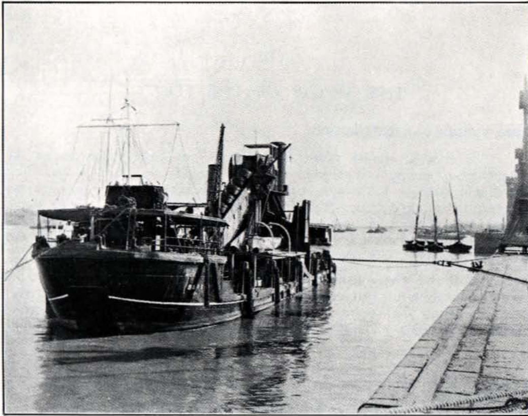
The Port Trust bucket ladder dredger " Barbus " at work off the Harbour Wall.
