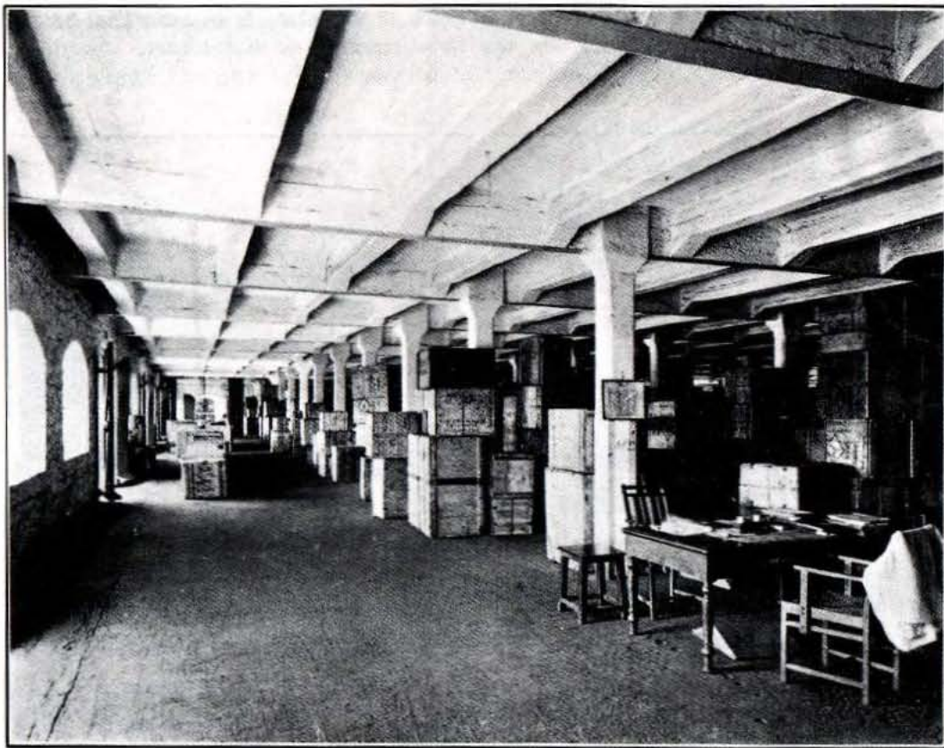
An upper floor interior, Alexandra Dock Warehouses.
