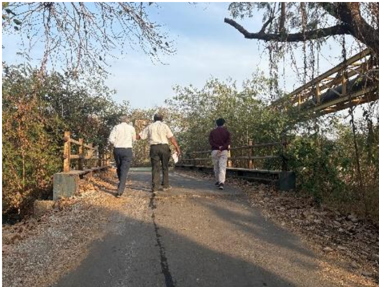
Figure 06: The bridge near the exit is approximately 4.5 m wide
